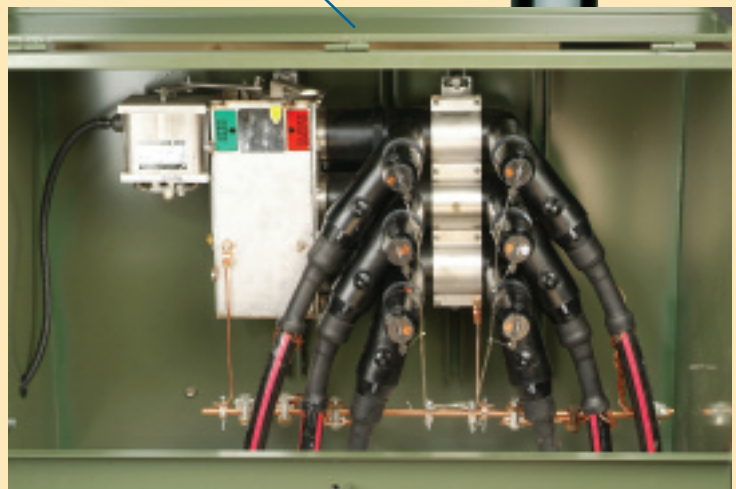
Motor Operated Switch
